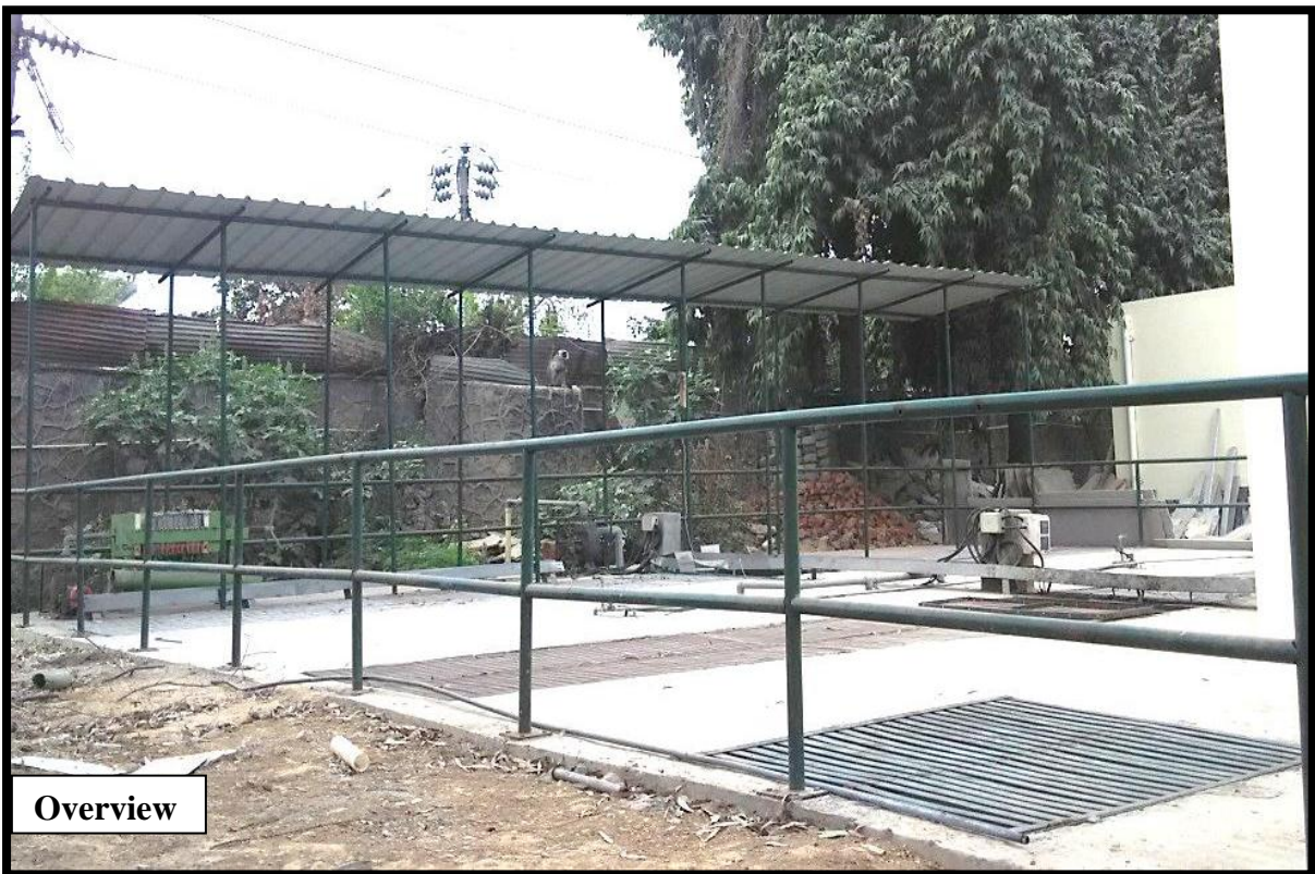
Effluent Treatment Plant
